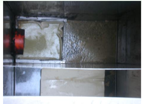
After > End Drainage Hole Is Clean
